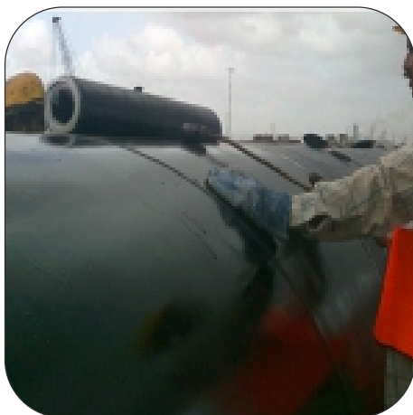
Ar Pipe Kote Bitumen Tape
